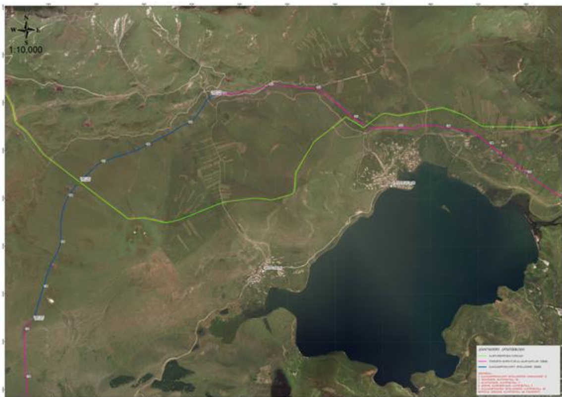
Figure 4.5. Rehabilitation section adjacent to Tabatskuri Lake
