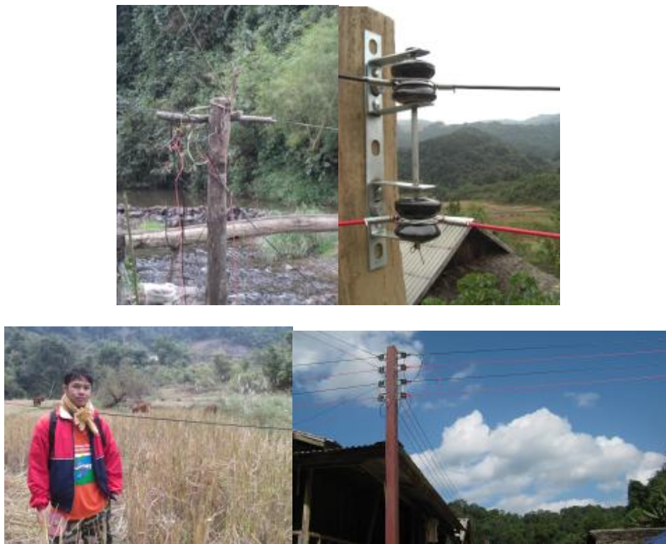
Figure 3: (Left Top & Bottom) Examples of previous bad wiring. (Right Top & Bottom) New wires provide a much safer and reliable system
