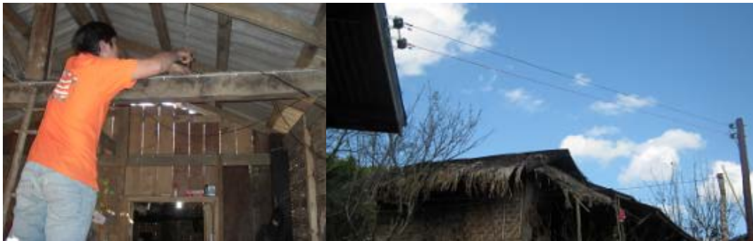
Figure 4: (Left) Showing old wires hanging loose (black) and new wires (grey) neatly pinned against beam. (Right) New household connection from power poles, using suspension clamps and steel rack
