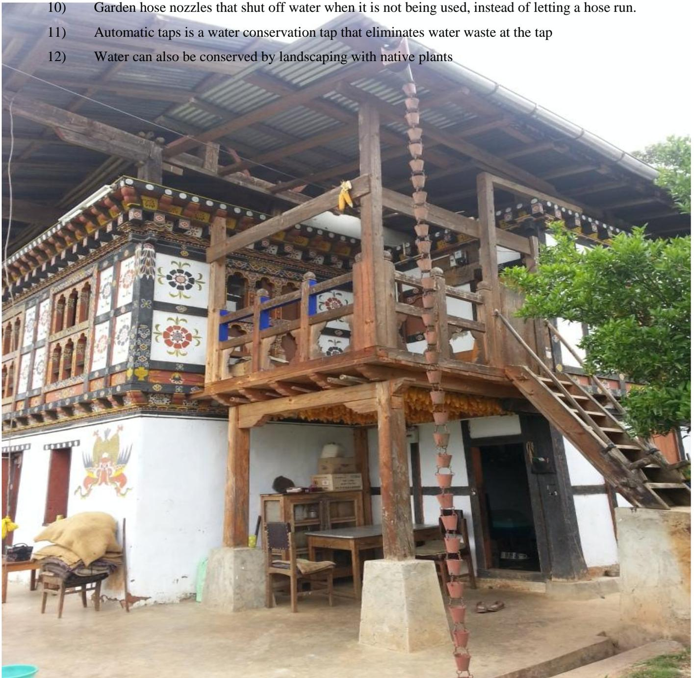
Rain water collection chains used in a house in Punakha
