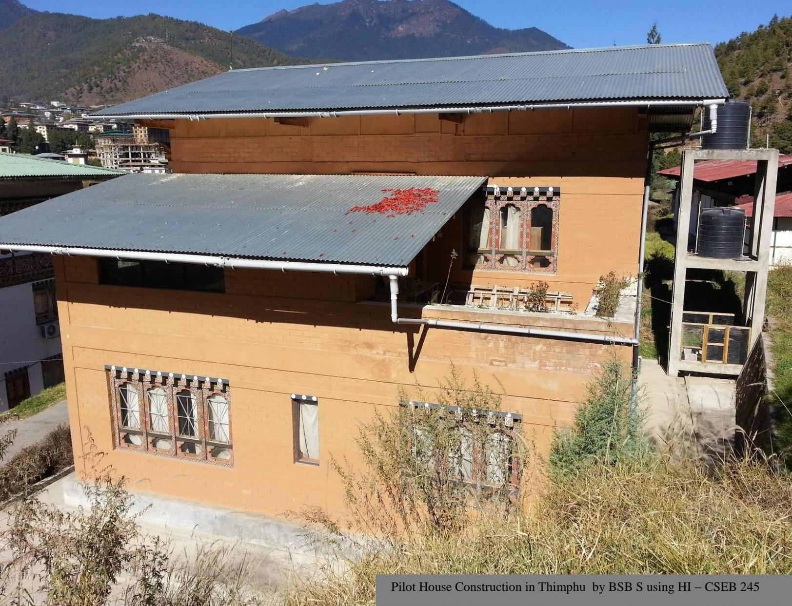
Pilot House Construction in Thimphu by BSB S using HI – CSEB 245
