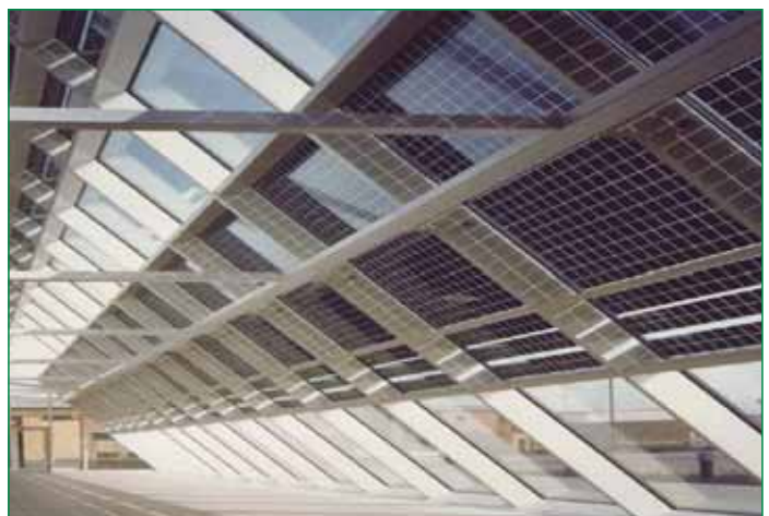
Fig (3) Building interior view 4
