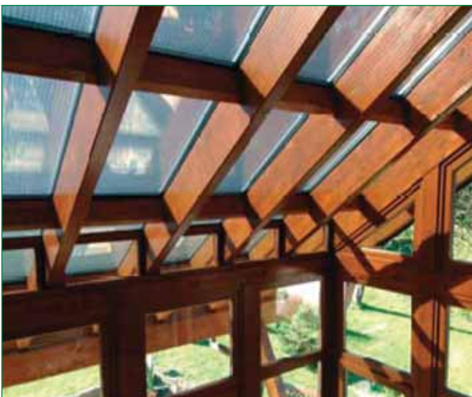
Fig (9) Building interior view 7
