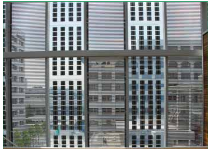
Fig (20) Building interior view 14
