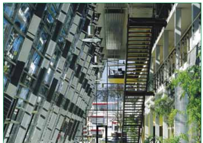
Fig (5) Building interior view 5
