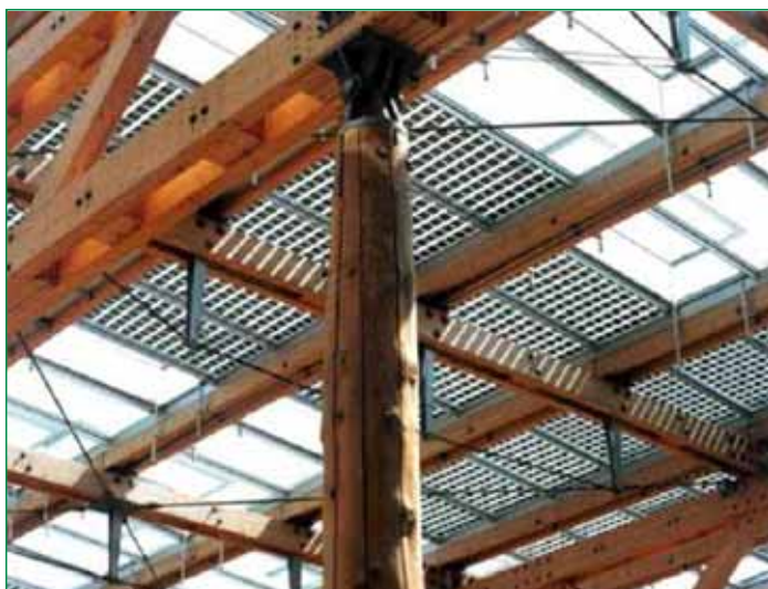
Fig (18) Building interior 13
