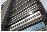
Sun-shading anti-glare – Control direct solar radiation
