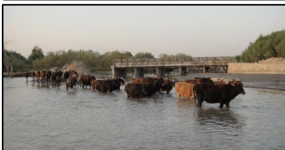
Before the implementation of the bridge project
