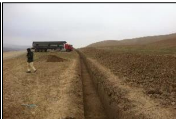
Photo: Excavation of the water supply trench system and installation of the HDPE pipe from Qadis district towards Qala – I – Now City | Photo Credit: RU-WatSIP © 2014
