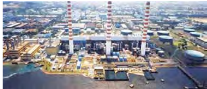
Aerial view of Senoko Power Station
