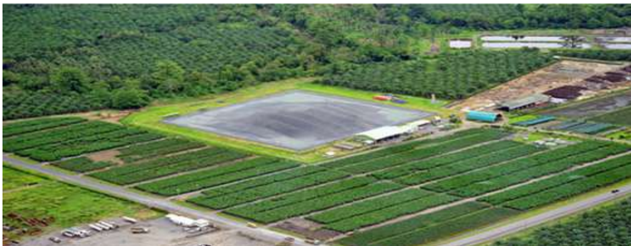
Figure 5. Biogas plant in New Britain Palm operation.
