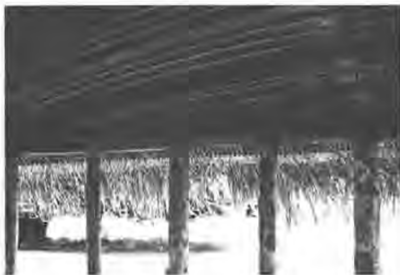
The new 'fale' at Samoa College, Apia, replaces the previous 'fale' destroyed by Cyclone Val. Built in traditional style, synthetic twine replaces the coconut sennet. (photo: A.C. Robinson, reproduced courtesy of DLSE)
