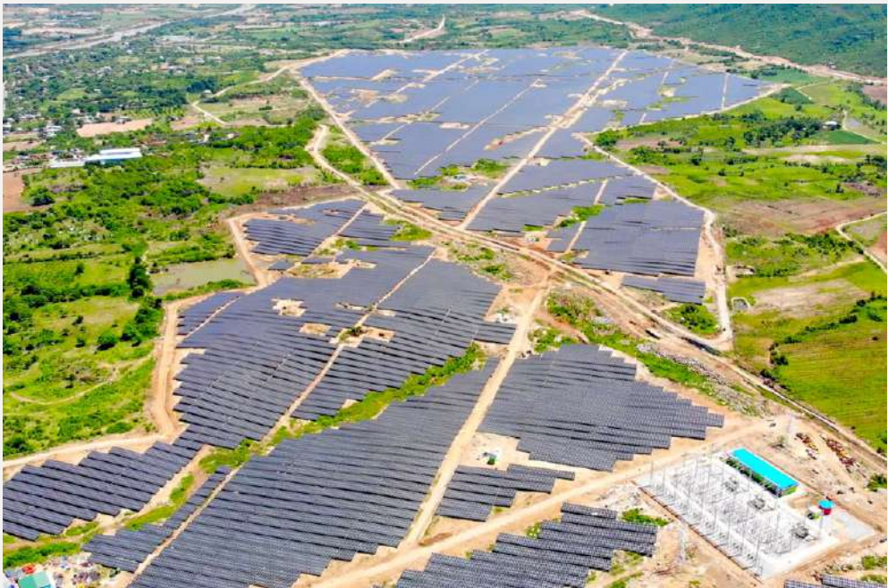
Sunseap’s 168 MWp solar farm in Ninh Thuan, Vietnam is one of the largest in the country. Sunseap and InfraCo Asia contributed three billion Vietnamese dong ($173,749) to fund the construction of concrete roads surrounding the site. At peak construction period, the project created over 2,000 jobs, mostly for locals in the area.
