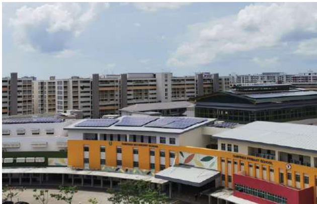
Tampines Secondary School is Singapore’s first positive energy school with several innovative energy-saving solutions such as vertical greenery, enhanced sunshades, smart fans and solar panels.
