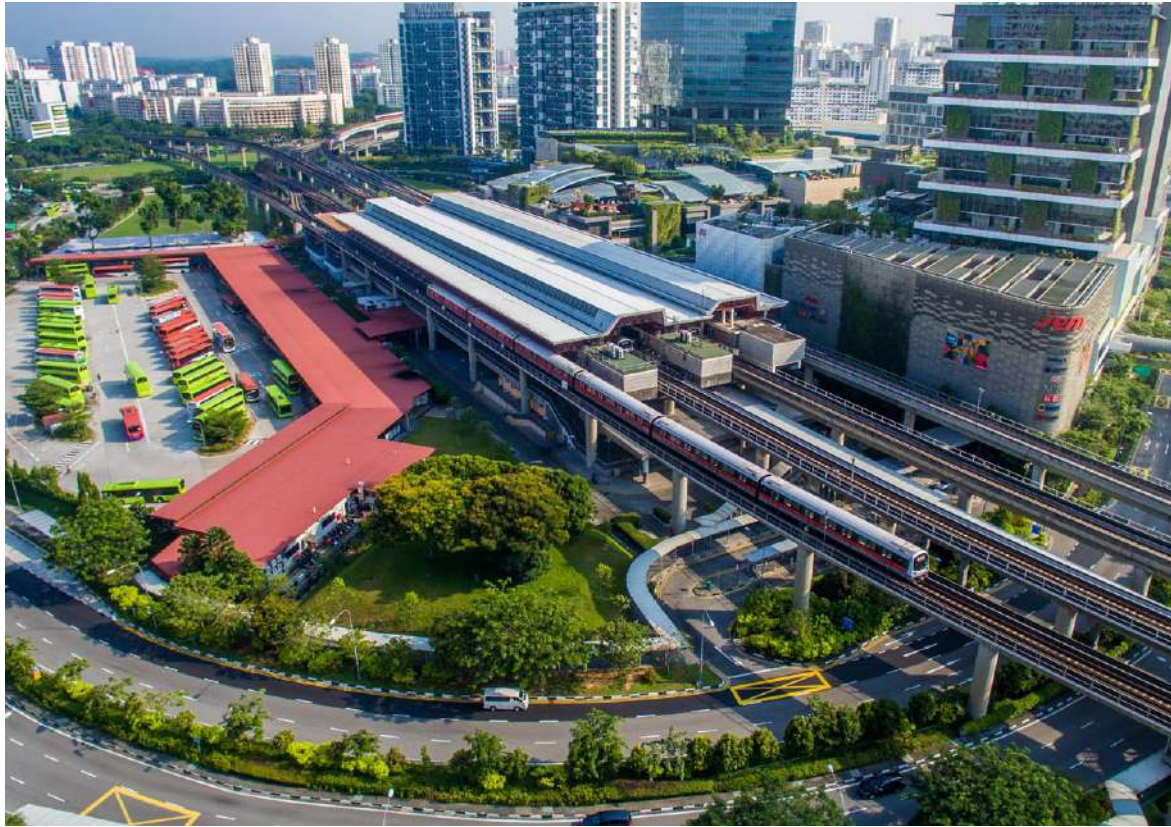
To encourage more people to take public transport, our public housing towns are designed such that their transport hubs integrate train stations with bus interchanges and are equipped with sheltered walkways that connect to housing blocks and amenities.
