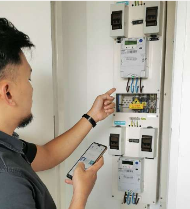
Advanced electricity meters enable households to track their half-hourly electricity consumption via the SP Utilities mobile app.
