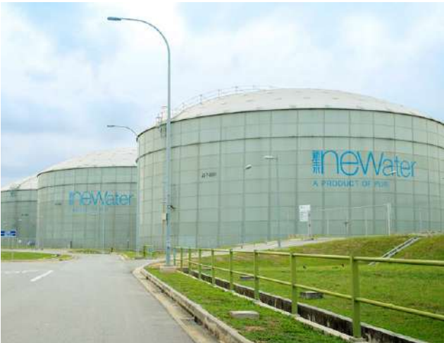
Singapore’s first NEWater plant, which is located in Bedok, began operations in 2002.
