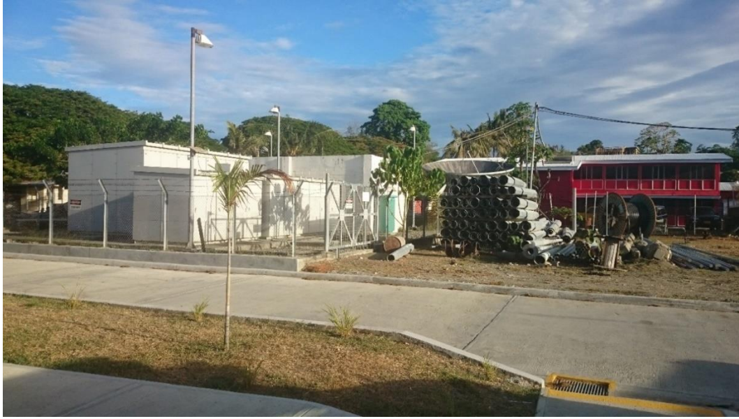
Ranadi Substation before upgrade
