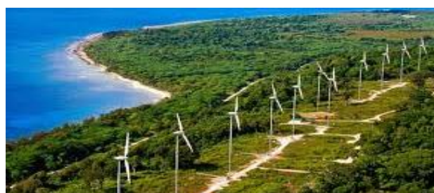
Devil's Point Wind Farm, Efate (3 MW)
