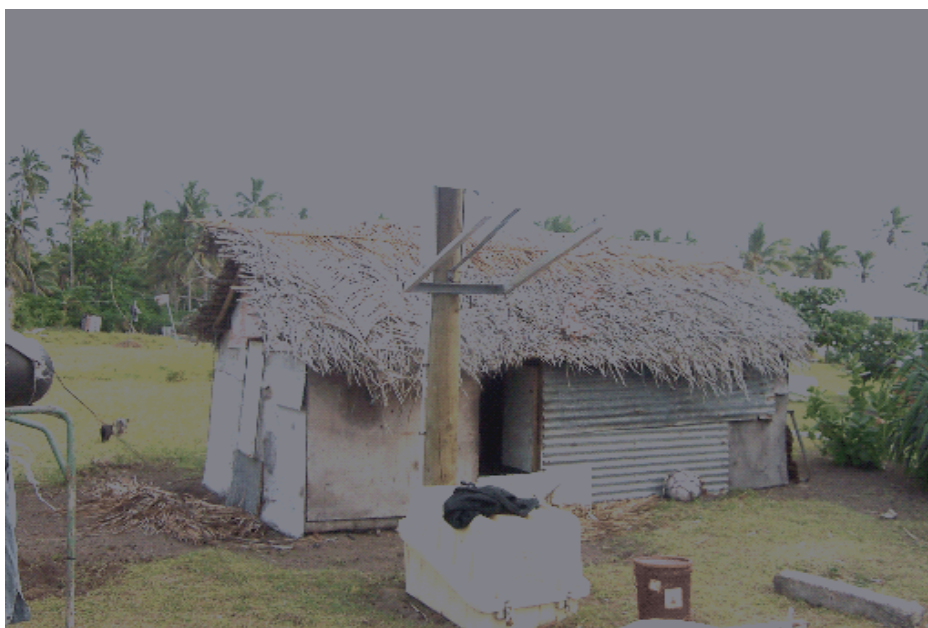
One of households electrified by Solar Energy in Fotuha'a Island, Ha'apai
