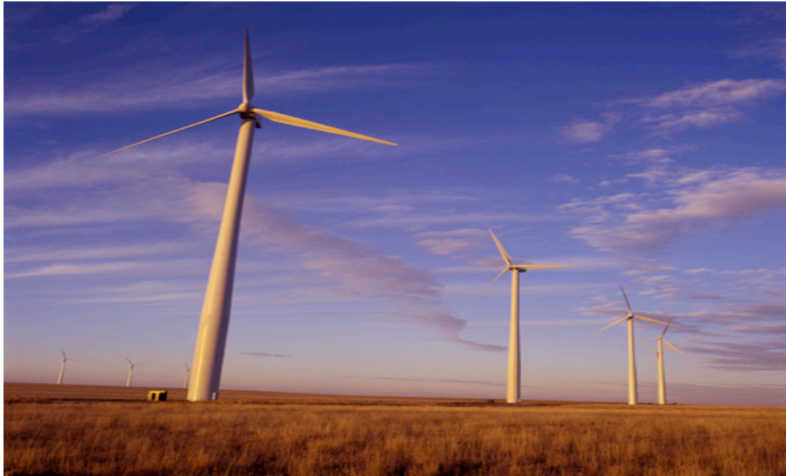
North America Wind Power Plant
