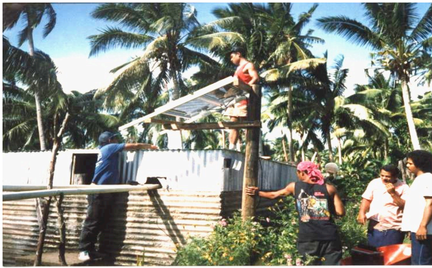
Installation of PV Systems in the Outer Islands...
