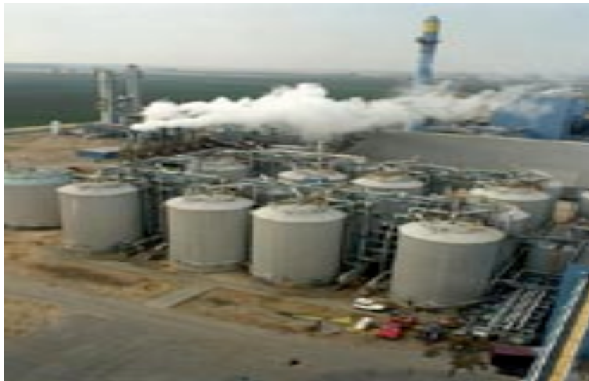
This generating station in Canada, burns biomass fuel from nearby sawmills produce energy.
